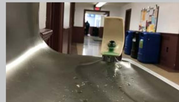
Above: According to studies, the blueish-green stains on water fixtures can be an indication of corrosion in the pipes.
